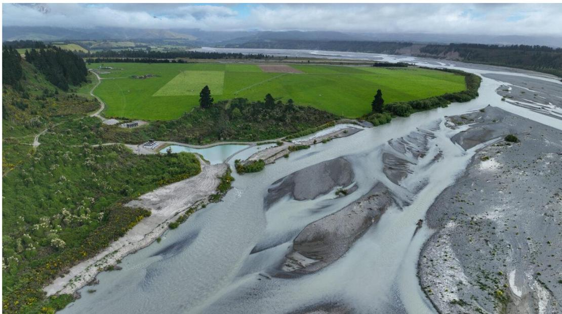
The below image shows the CPWL Rakaia River intake built with limited hard materials, to supply water Stage 1 and 2 of the Scheme. Of the 5.3 billion m3 of water that flowed in the Rakaia River over the past year, CPWL shareholders utilised 2.0% to grow food and fibre.
